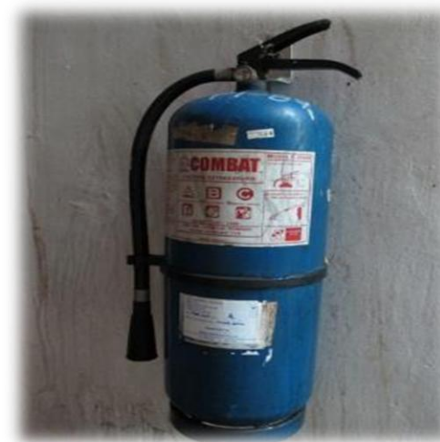
Fire Extinguishers expired, depleted or damaged
