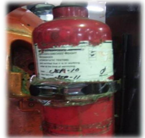
Fire Extinguishers expired, depleted or damaged
