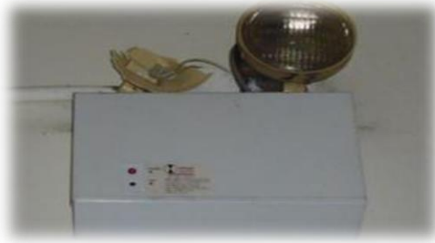
Exit Lights & Emergency Lights Malfunctioned / Damaged
